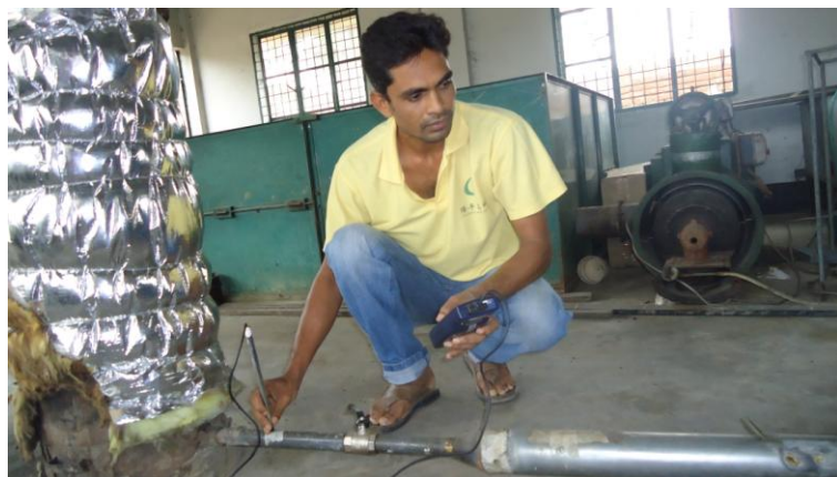
Fig.4.1.5: Measurement of Air velocity in the air inlet pipe
