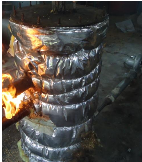
Fig.4.1.1: Combustible gas burning by firing
